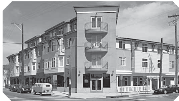
Sacramento Street Senior Homes, Berkeley, California
